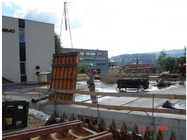
Dalle sur parking
